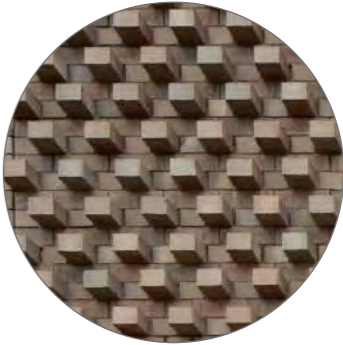
2. Contemporary brickwork features
