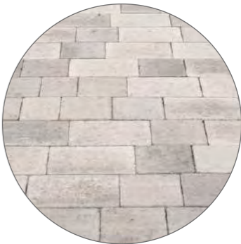
6. Resurfaced vehicular access with permeable paving
